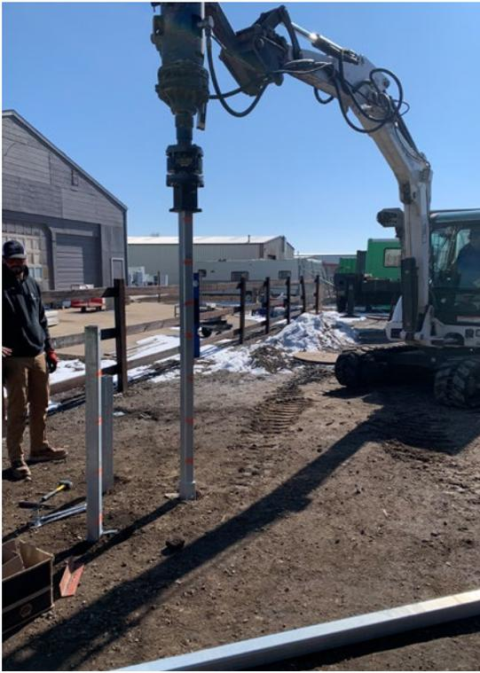
1. Alignment and installation of helical piers
