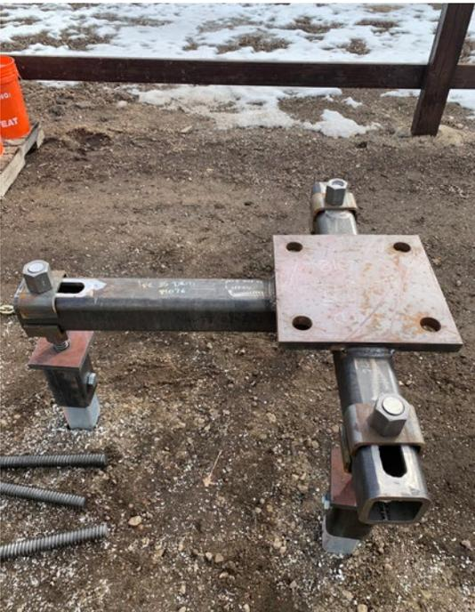
3. Adapter component connected to pier caps
